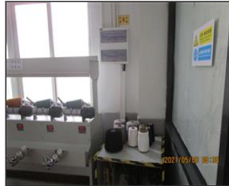
Photo of non-conformity NC-Electrical switches were blocked.JPG
