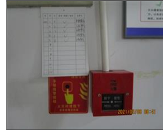
Photo of fire safety equipment Fire alarm.JPG
