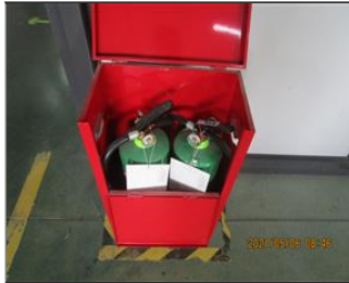
Photo of fire safety equipment Fire extinguishers.JPG
