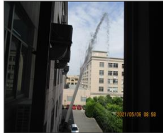
Photo of fire safety equipment Hydrant test.JPG
