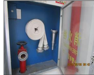
Photo of fire safety equipment Hydrant.JPG
