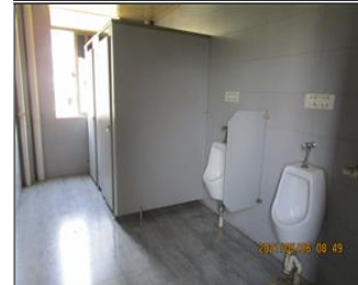
Photo of the sanitary facilities Toilets.JPG
