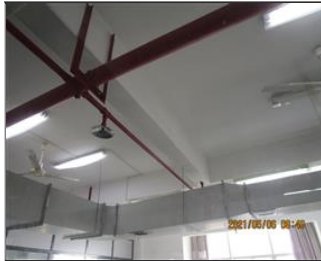
Photo of fire safety equipment Sprinkler.JPG
